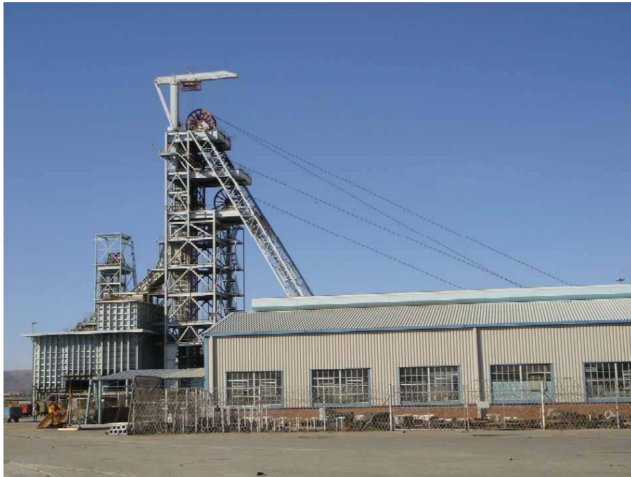
Figure 1: Karee No. 3 Main Shaft headgear, the top two ropes are the rock winder ropes.
